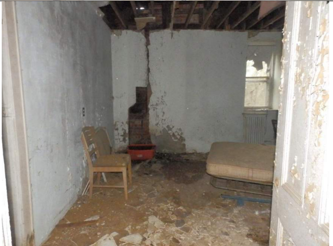
72. Room 301, looking west.
