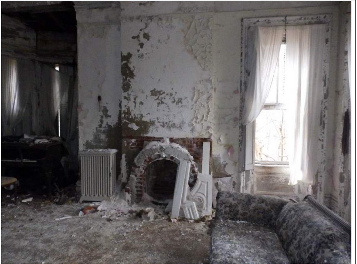
50. From Room 105, looking west into Room 101.0
