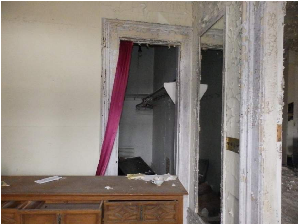
49. Room 105, looking south.
