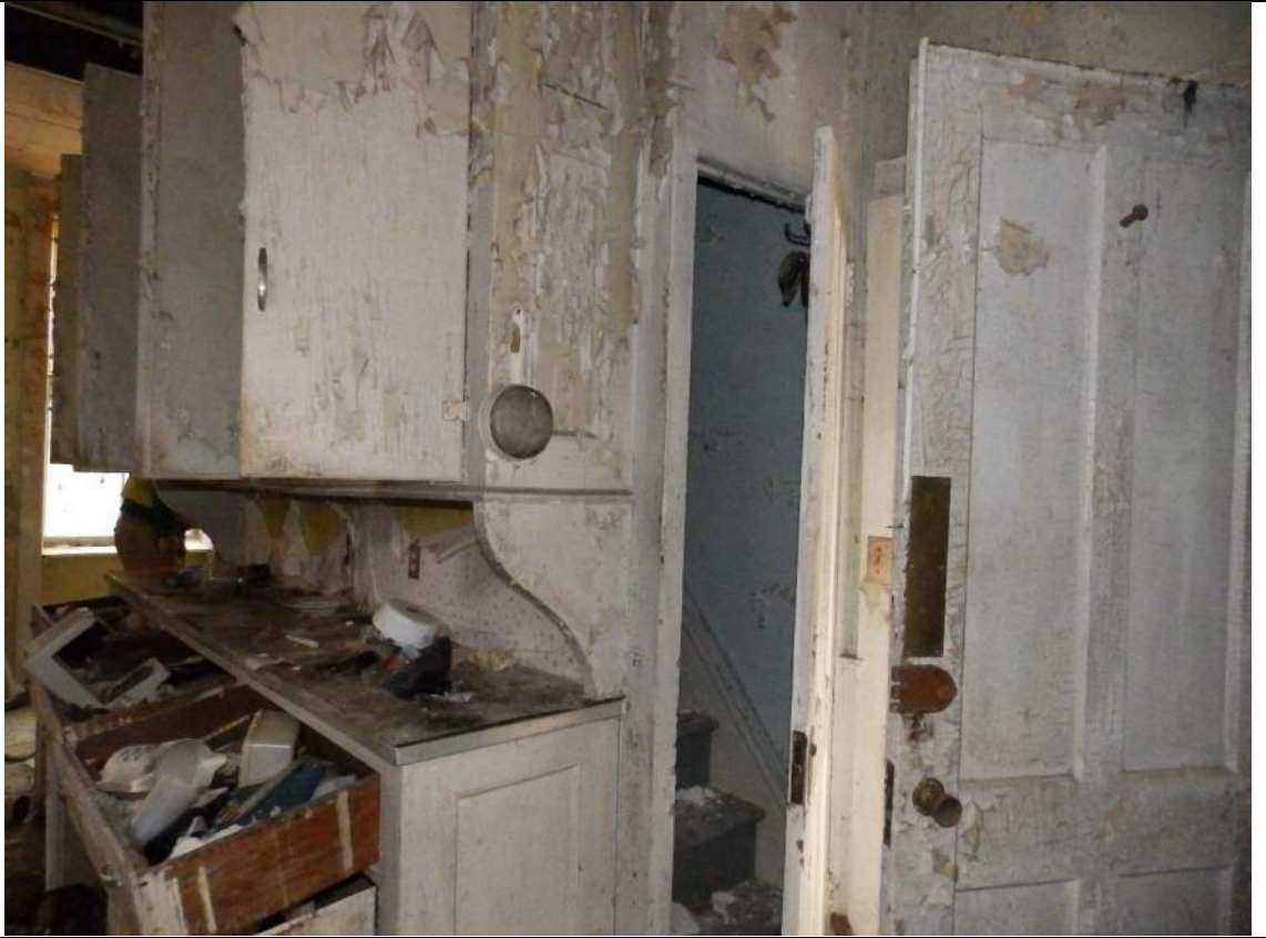
43. Room 106, looking southwest.
