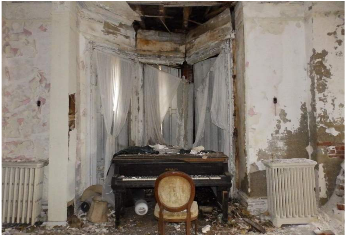
32. Room 101, looking west.
