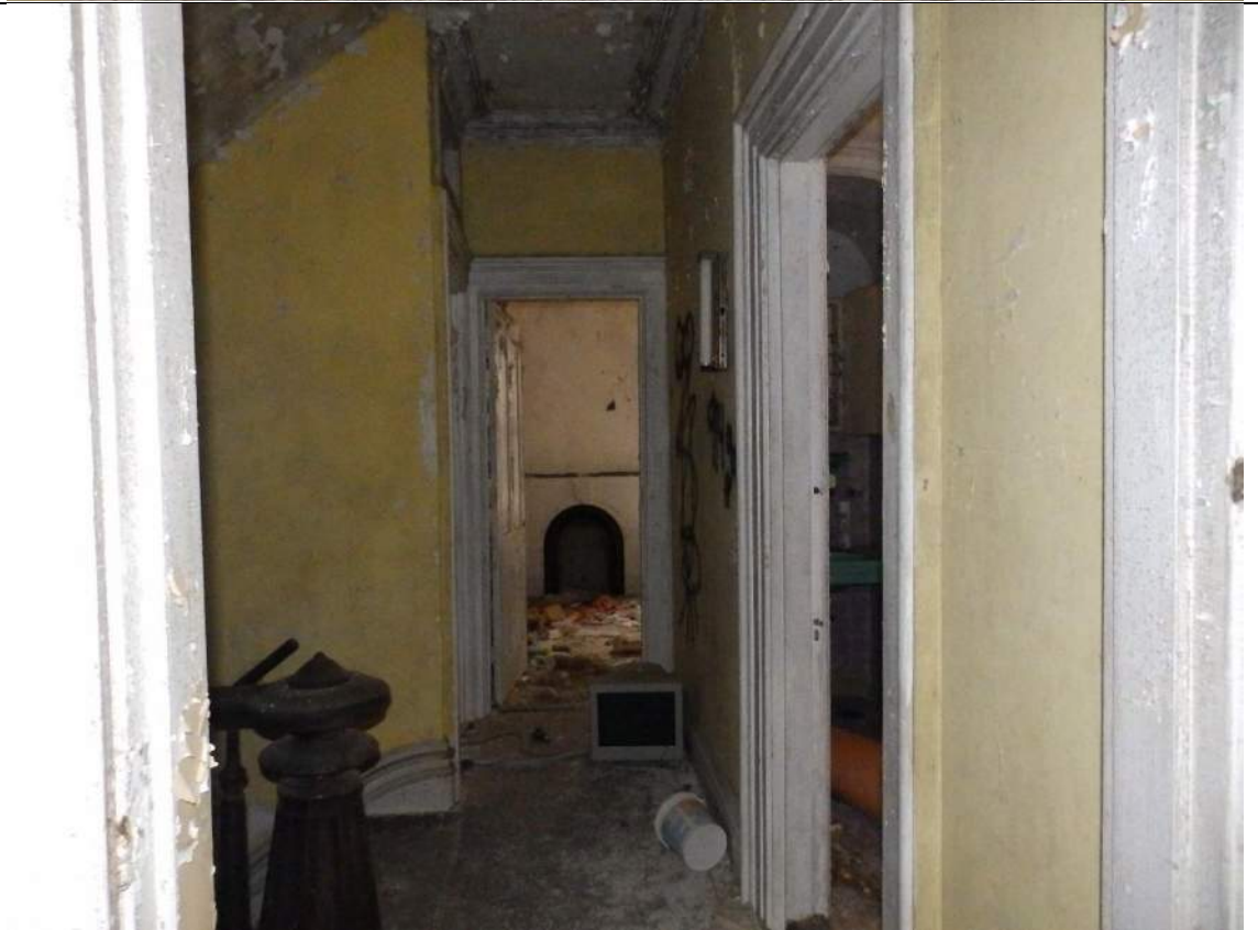
52. Second floor hall, looking east.
