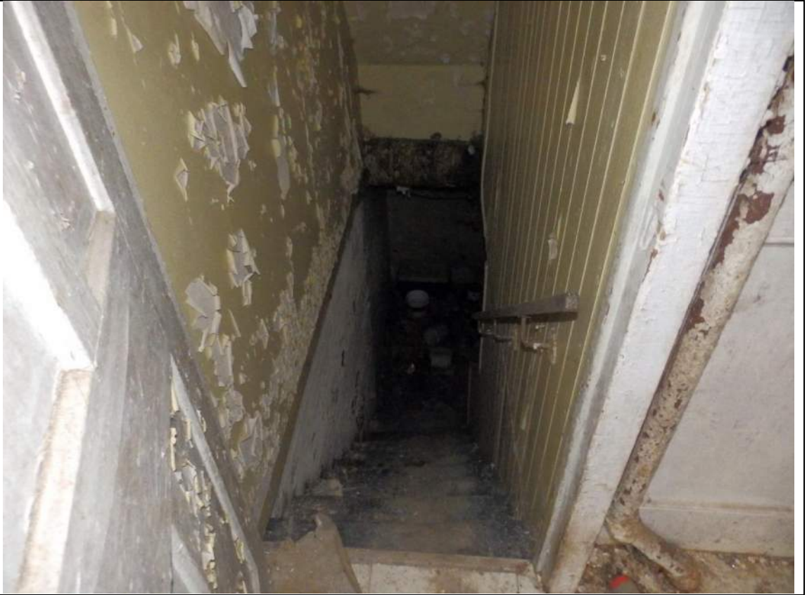
45. Stairs to the cellar, looking west.
