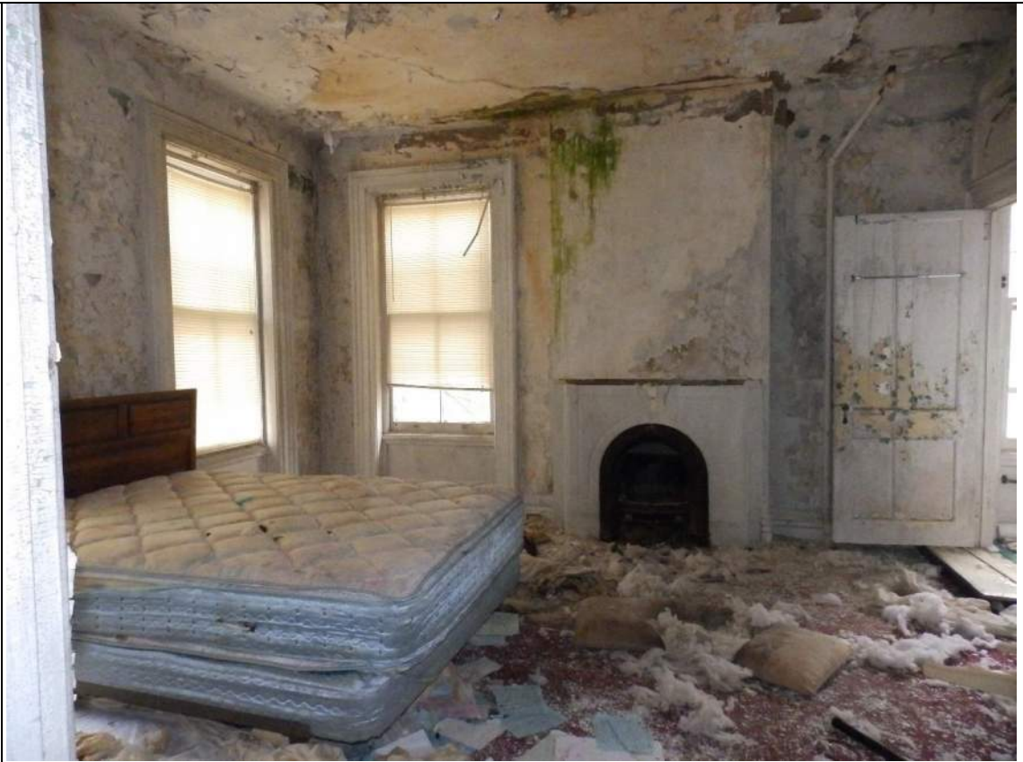
57. Room 203 looking west.
