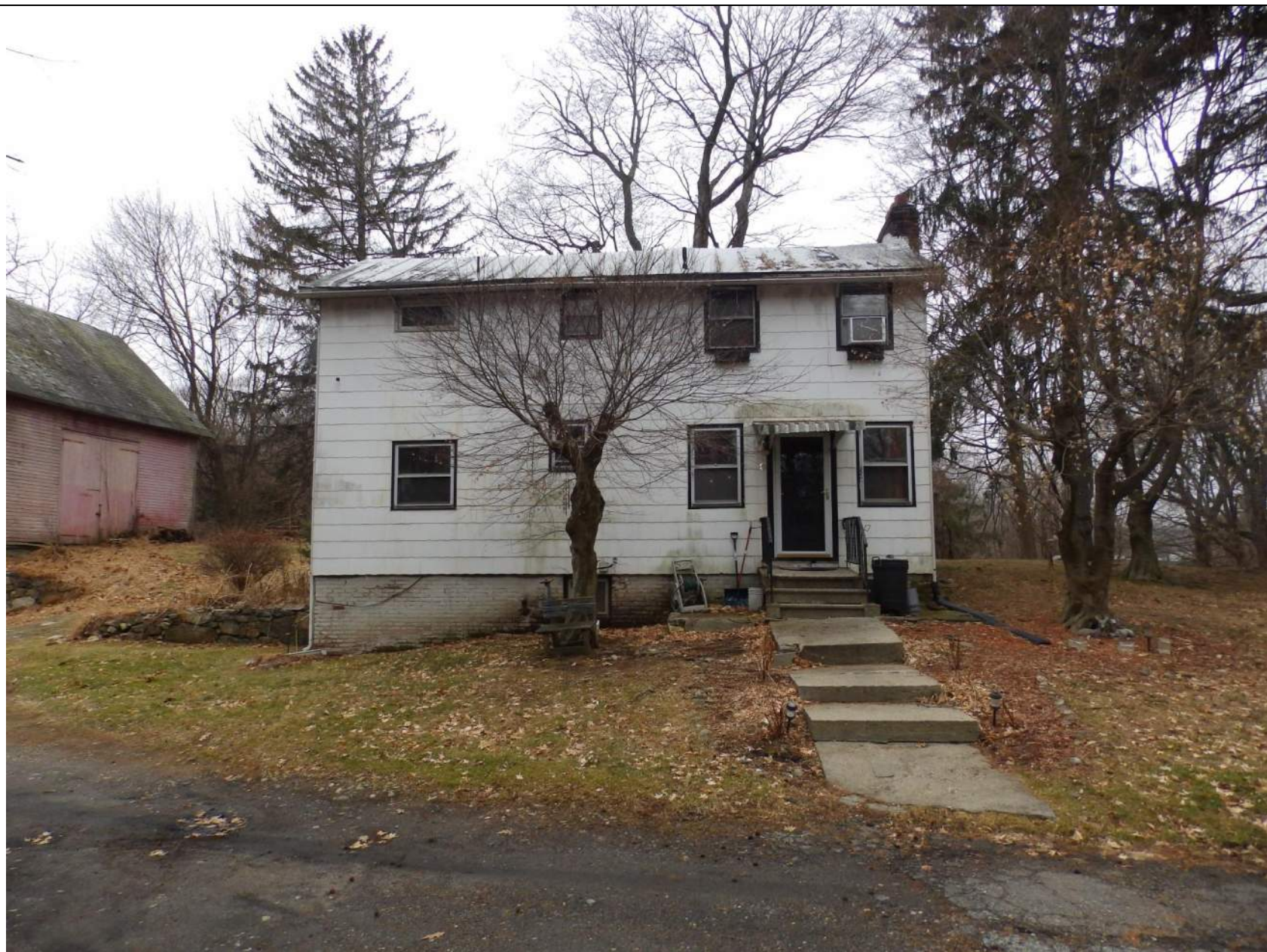
26. View of the façade of the caretaker's house.
