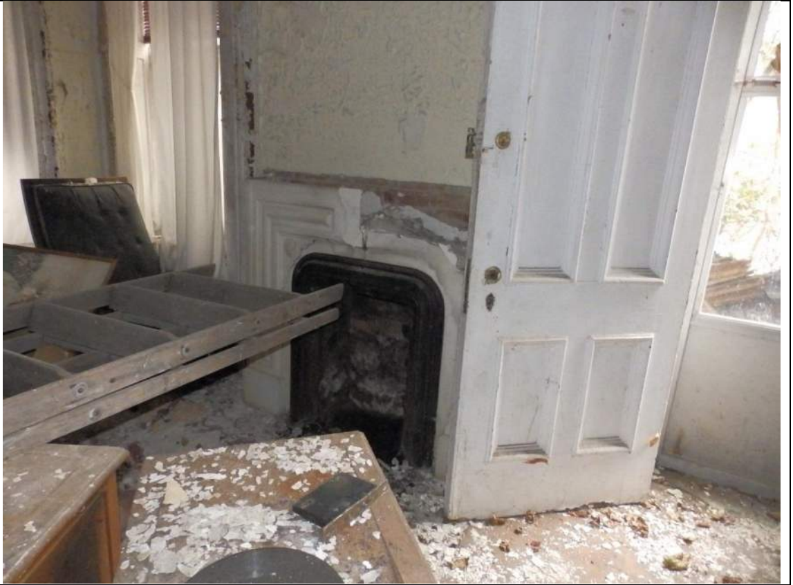
47. Room 104, looking east.
