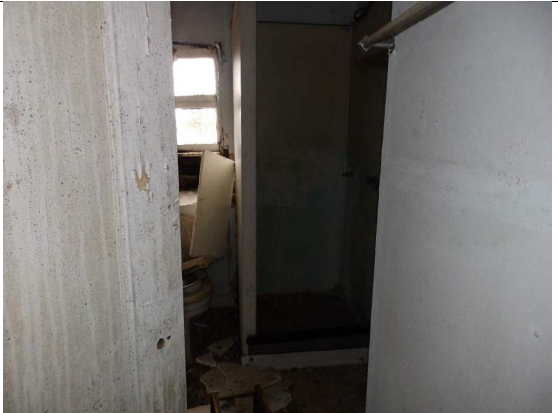
85. Room 309, looking north.
