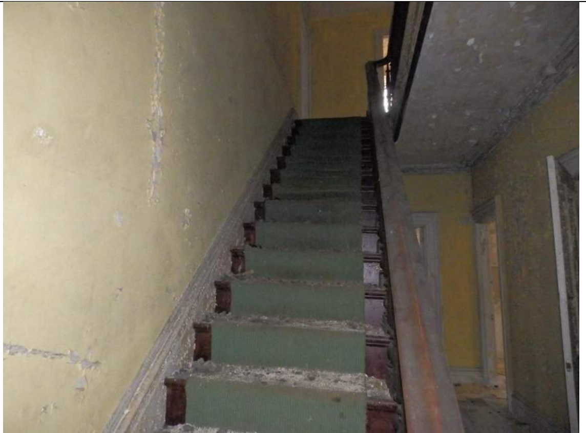
69. Stairs to the third floor.
