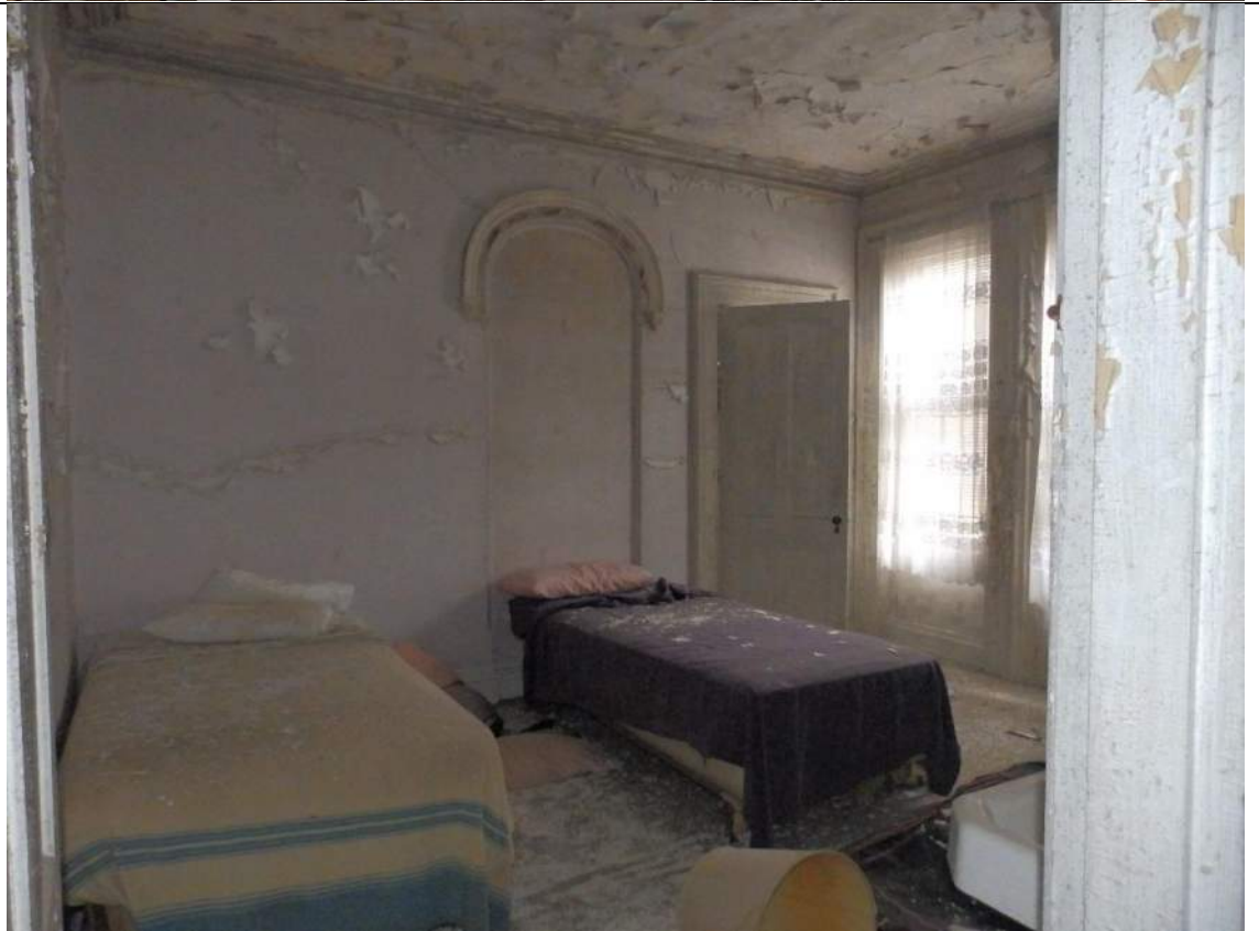
64. Room 209, looking southeast.
