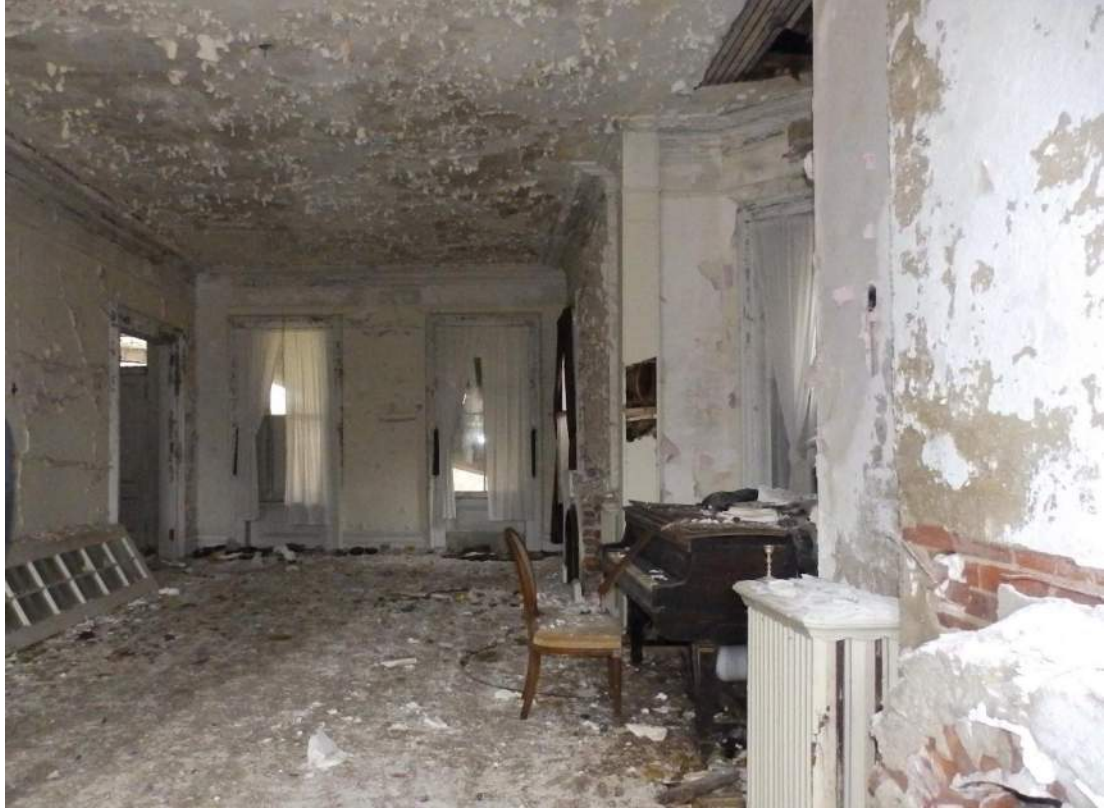
31. Room 101 looking south.
