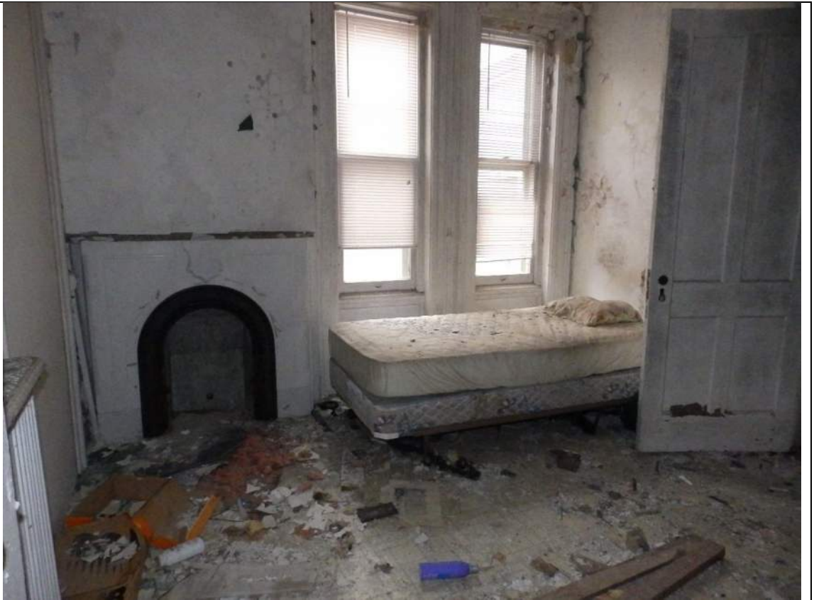
61. Room 205, looking east.
