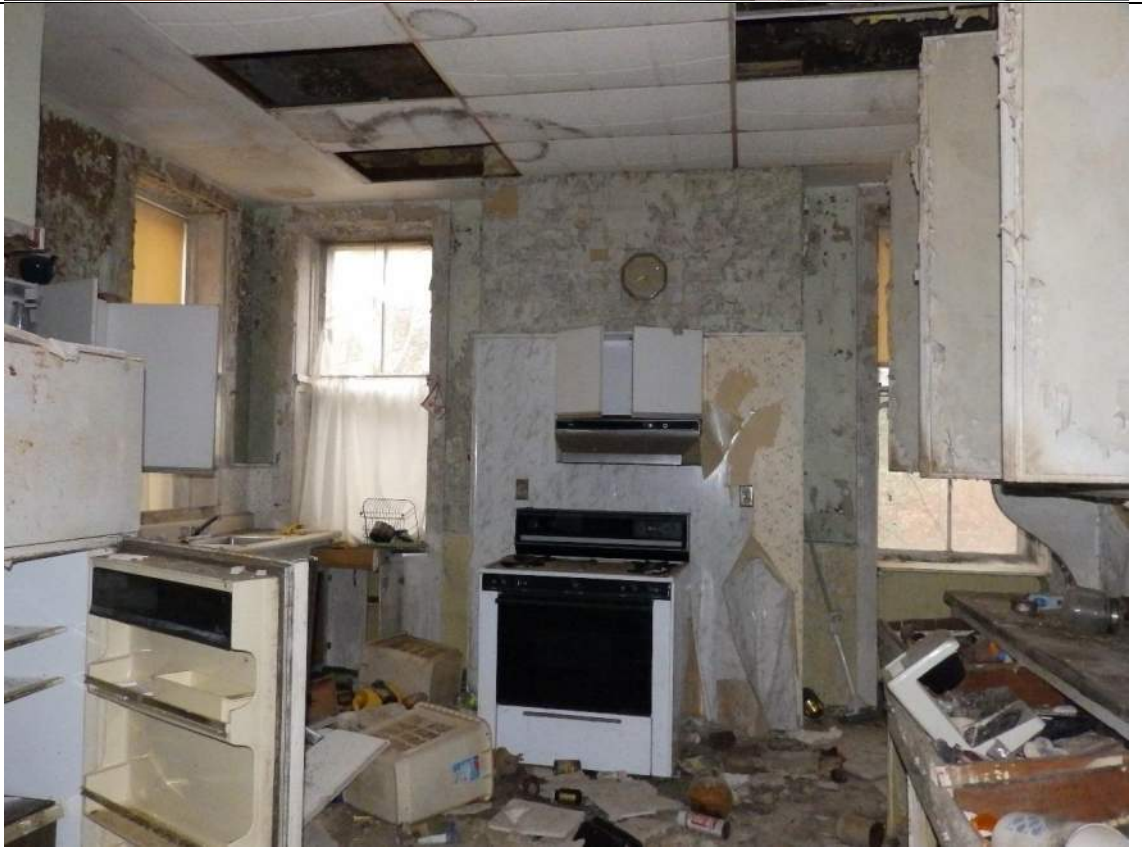
40. Room 106, looking south.
