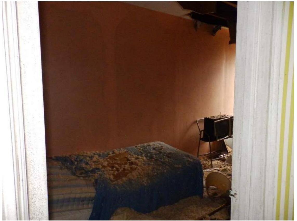
79. Room 306, looking east.
