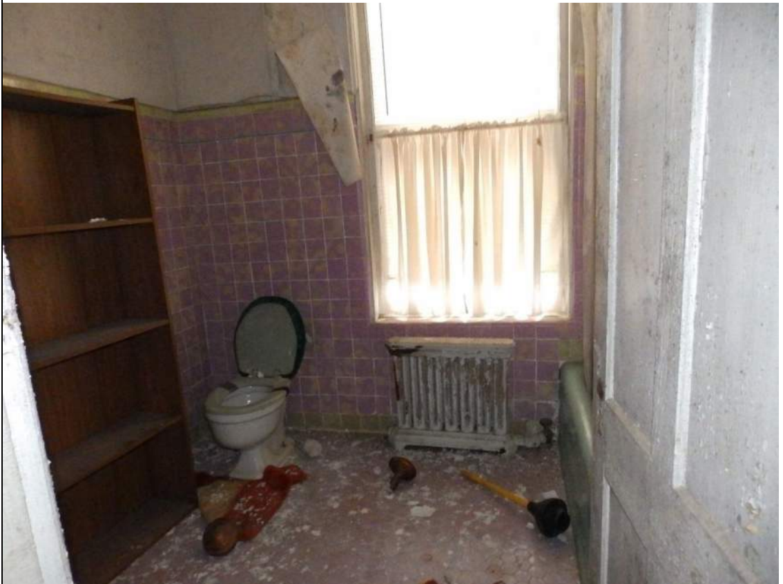
60. Room 204, looking south.
