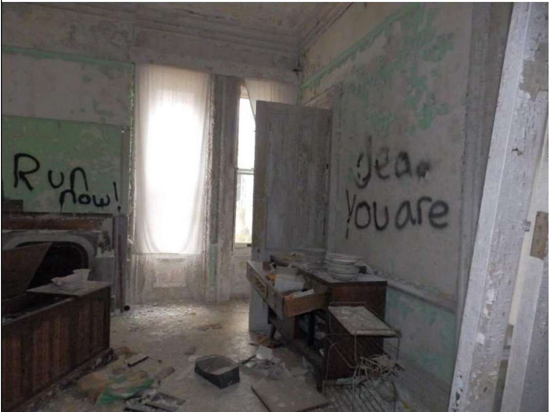
36. Room 103, looking east.
