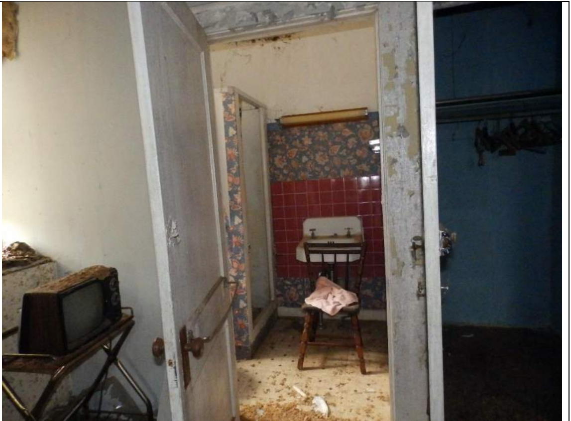
75. Room 302, looking north.
