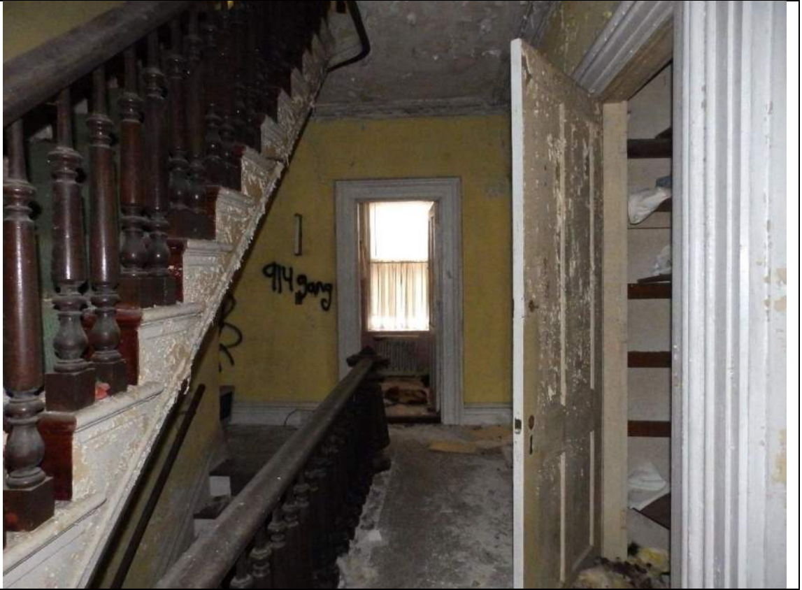
54. Second floor hall looking south.
