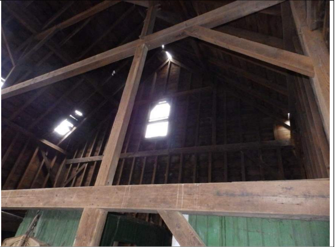
87. Upper space on the western side of the barn.
