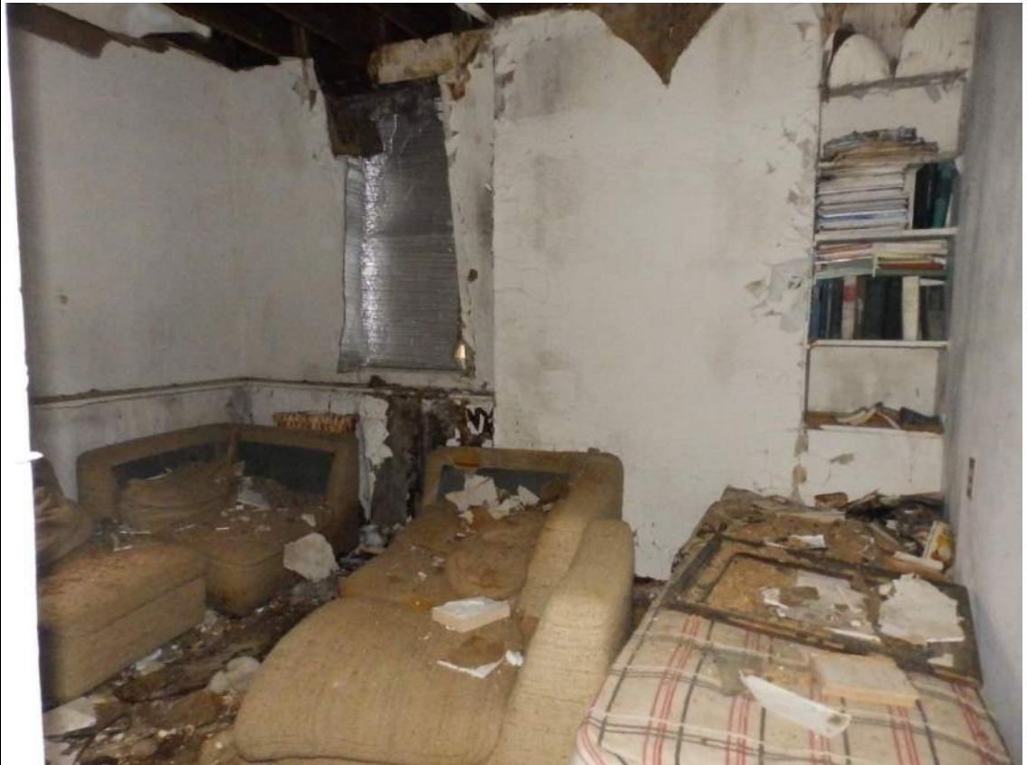
82. Room 308, looking east.
