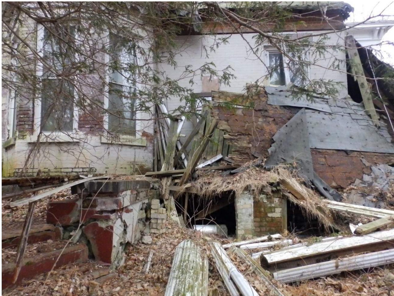
6. Detail of patio and cellar entrance on western elevation.
