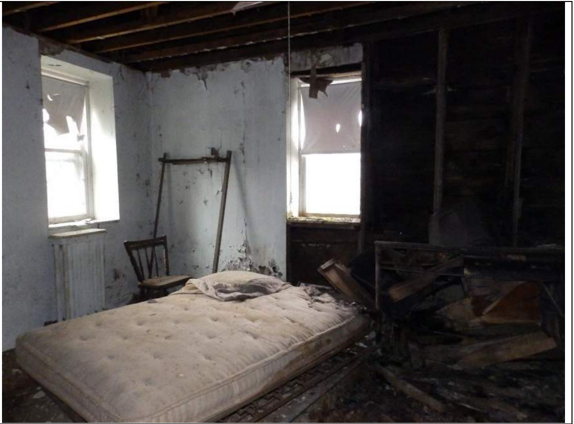
73. Room 301, looking north.
