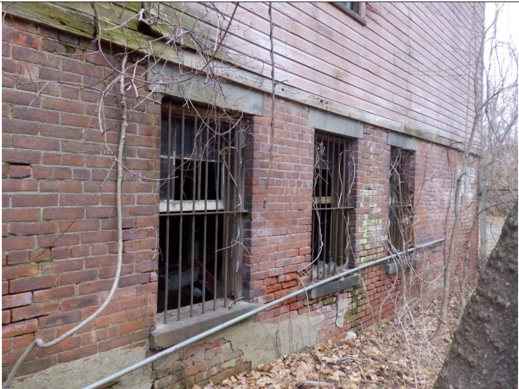
20. Detail of the openings to the former horse stalls.
