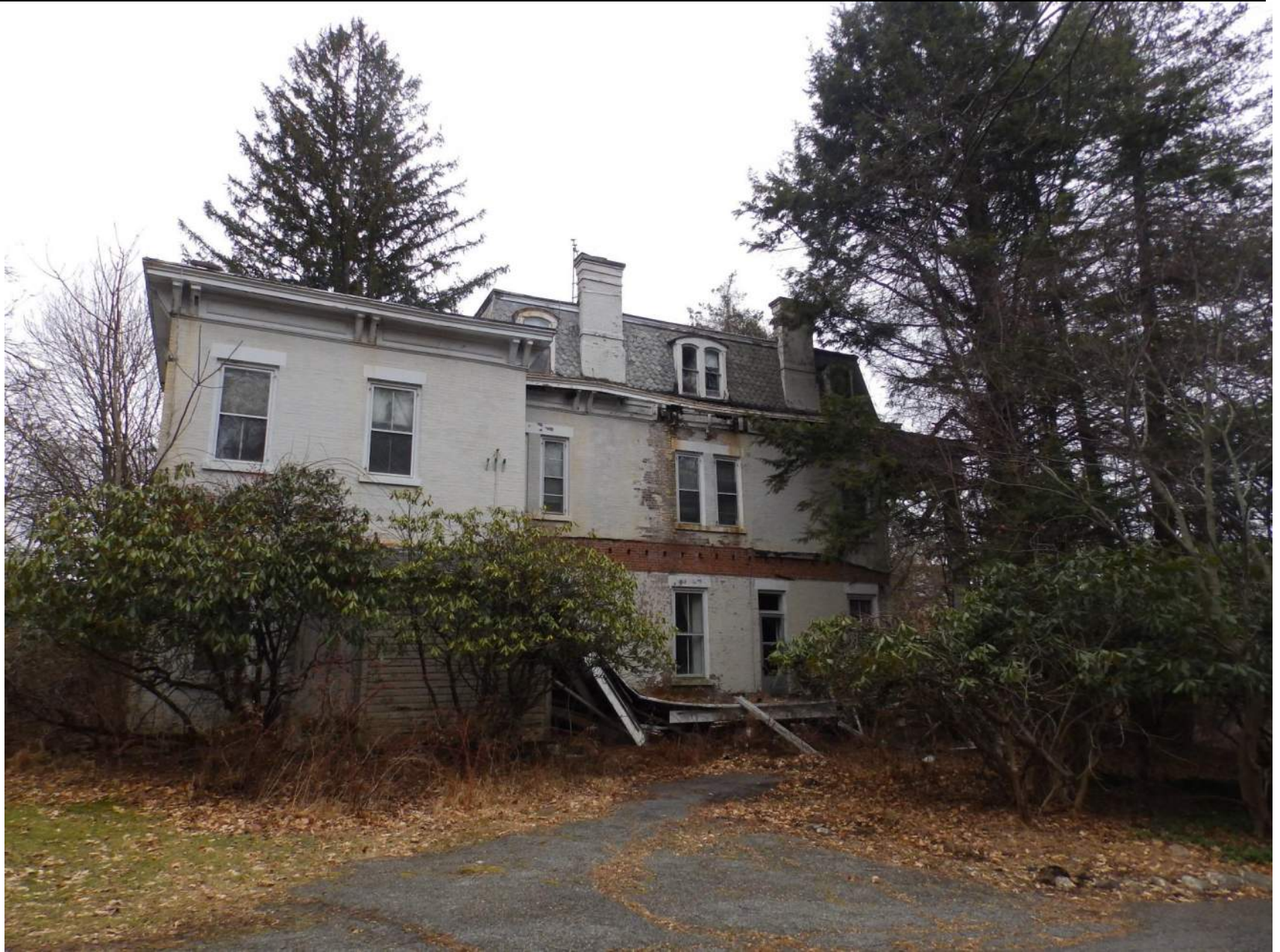
7. Evergreen Manor eastern elevation.
