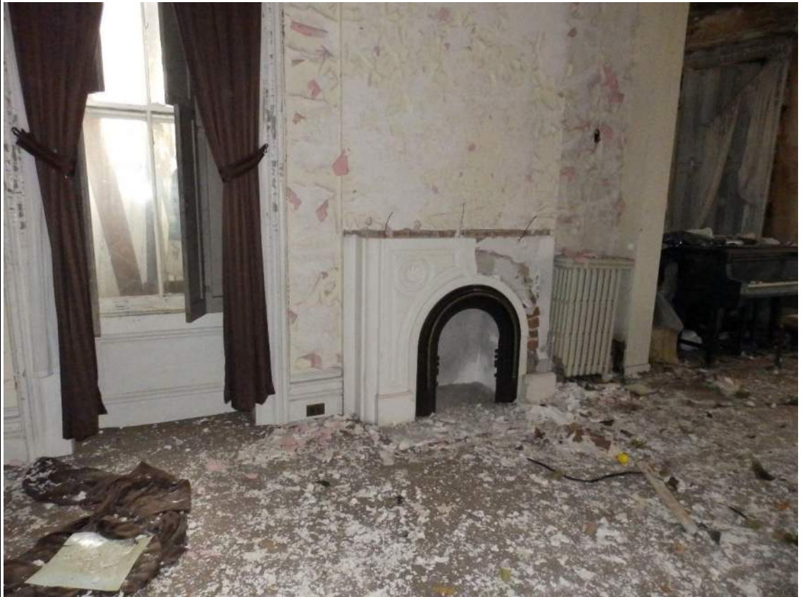
34. Room 101 looking northwest.
