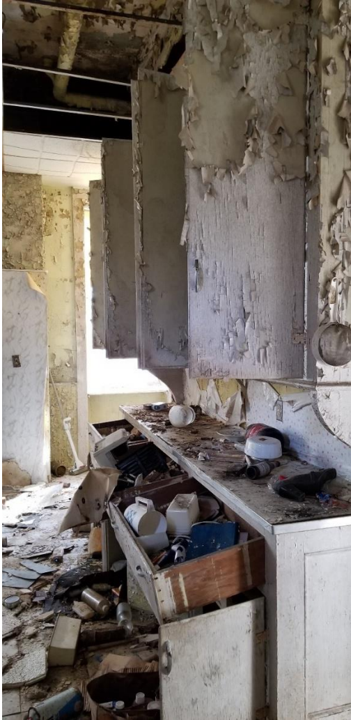
25. Kitchen – renovated after construction of structure
