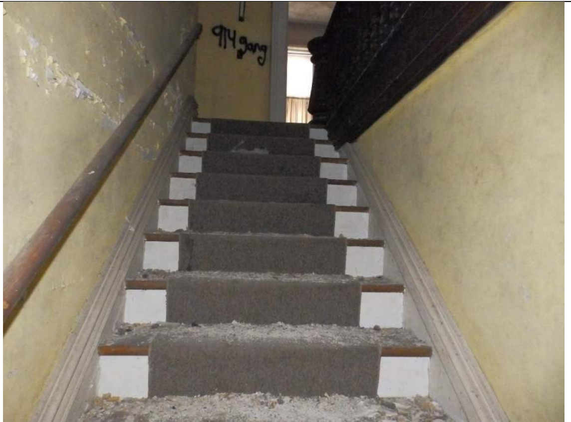
51. Stairwell to the second floor.
