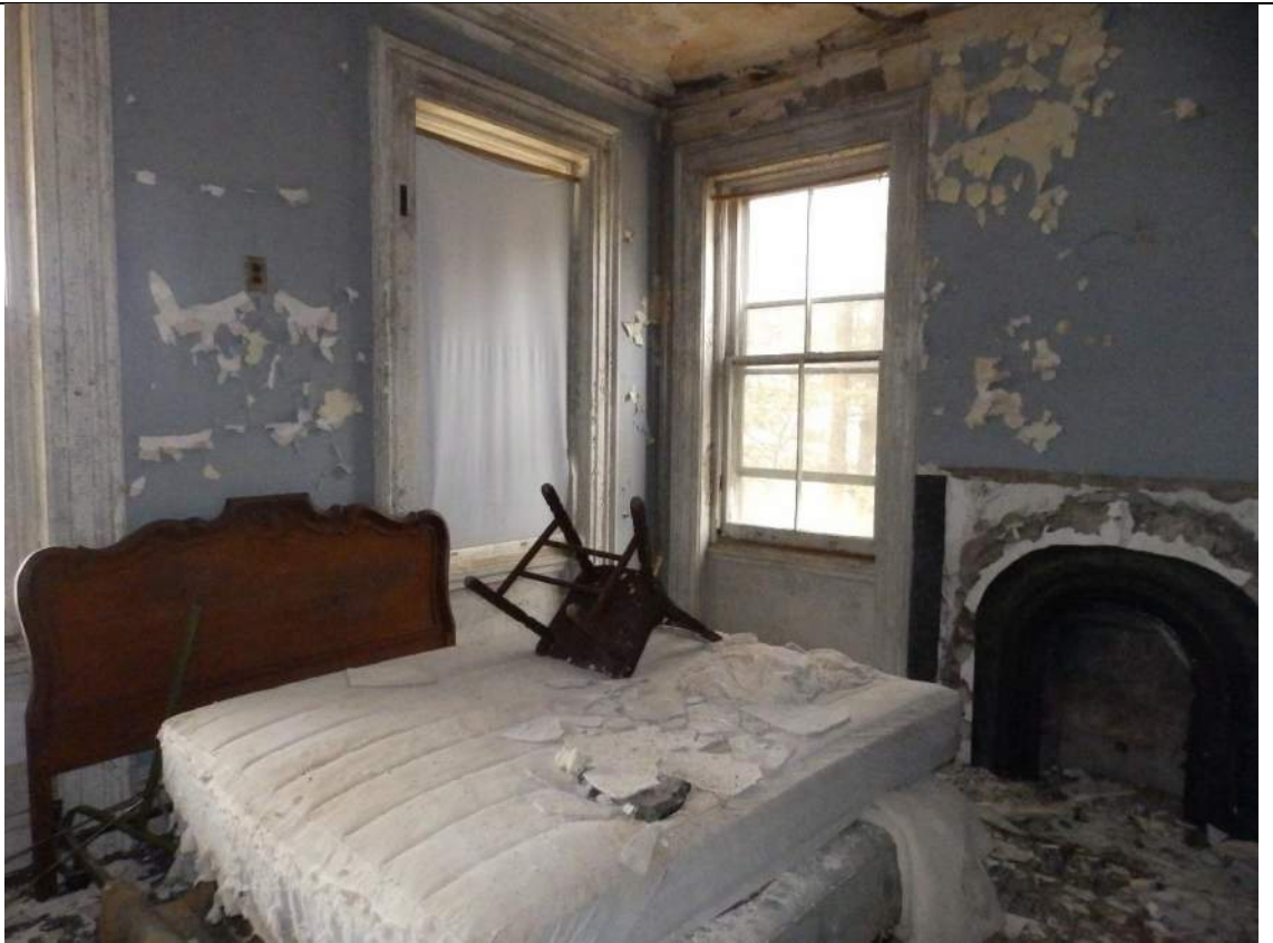
67. Room 210, looking northeast.
