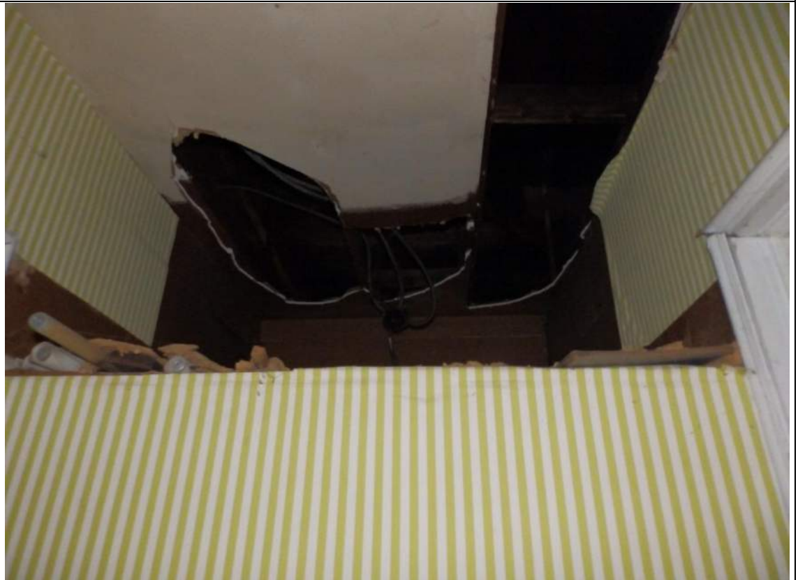
80. Storage area between Rooms 305- 306.
