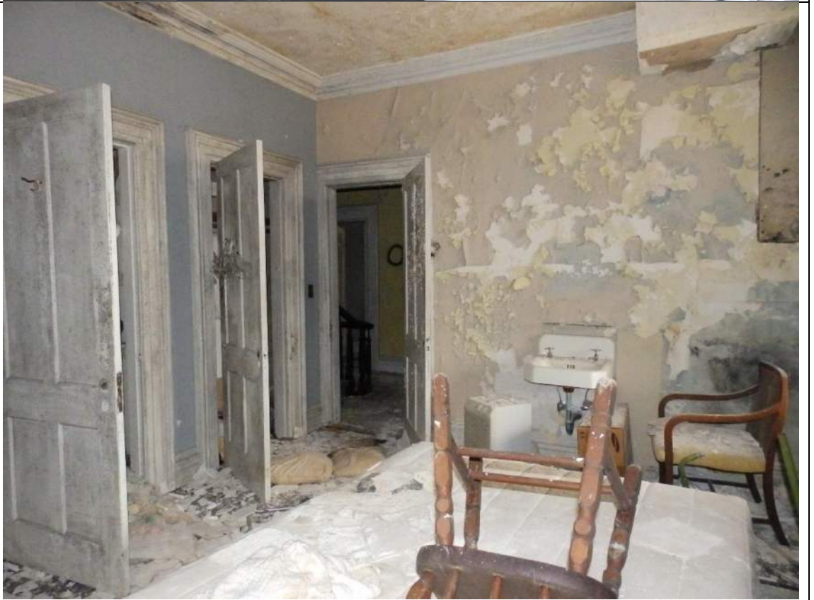
66. Room 210, looking west.
