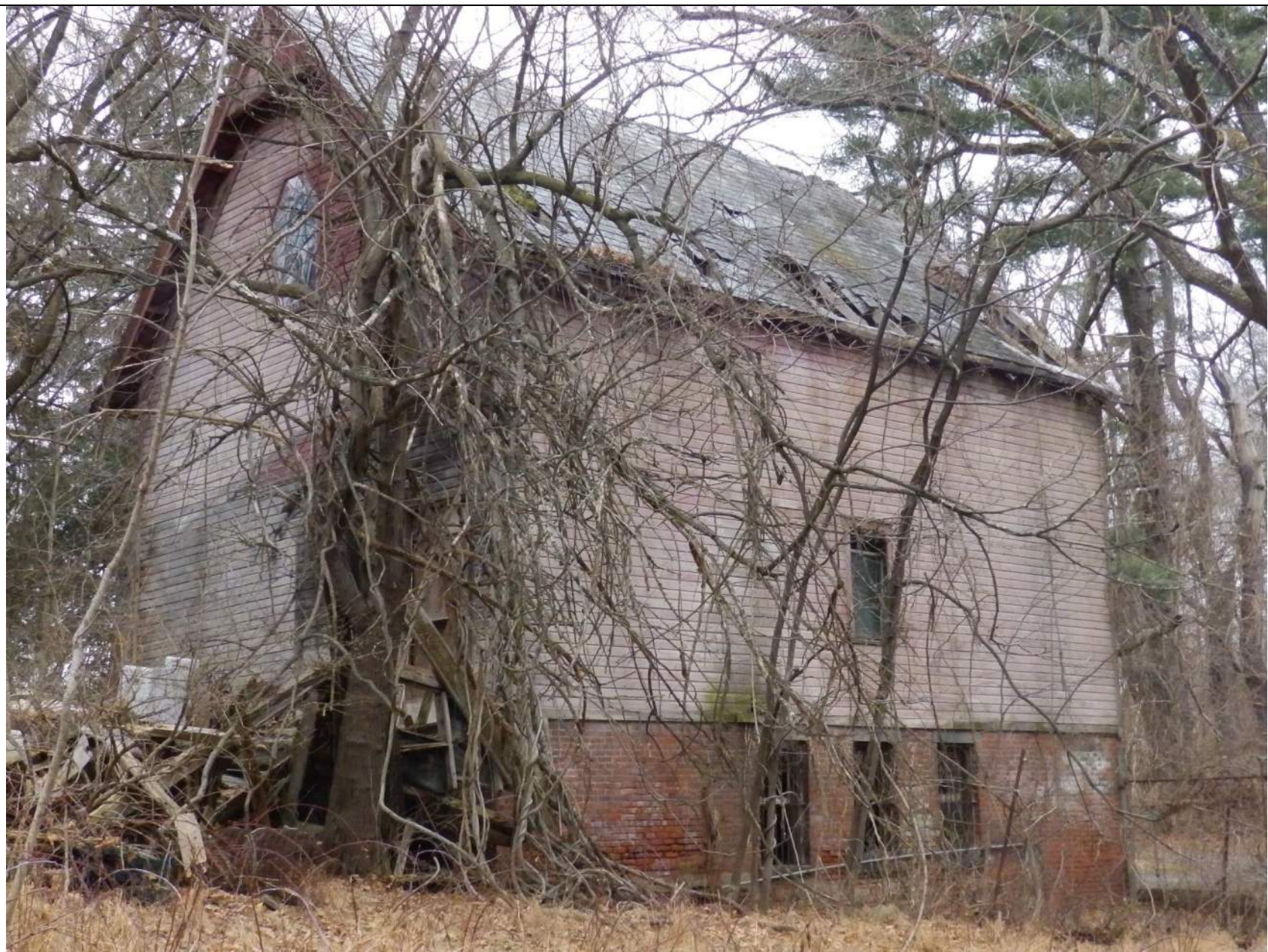
18. Oblique view of the western and southern elevations of the barn.
