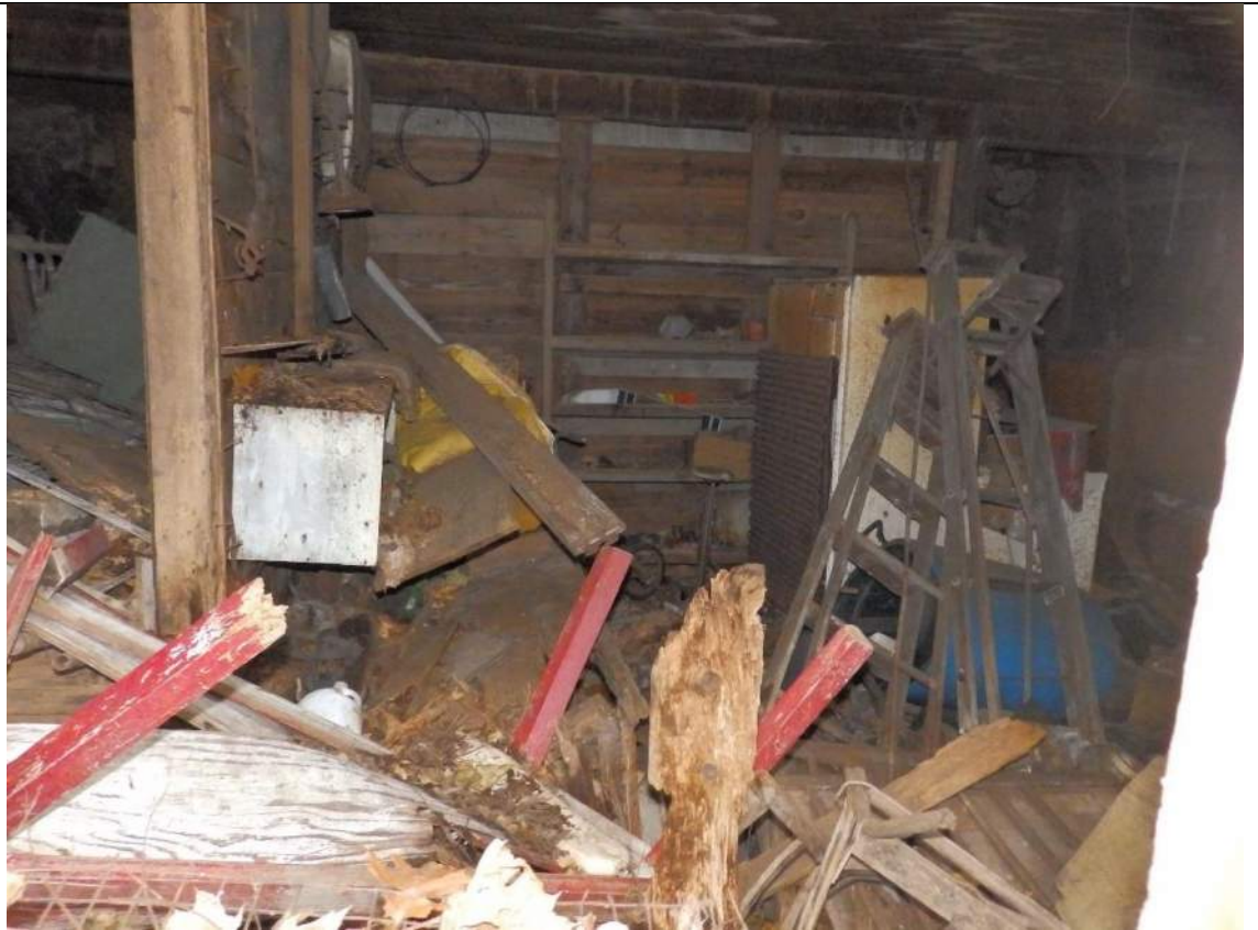
89. Lower level of the barn, looking east.
