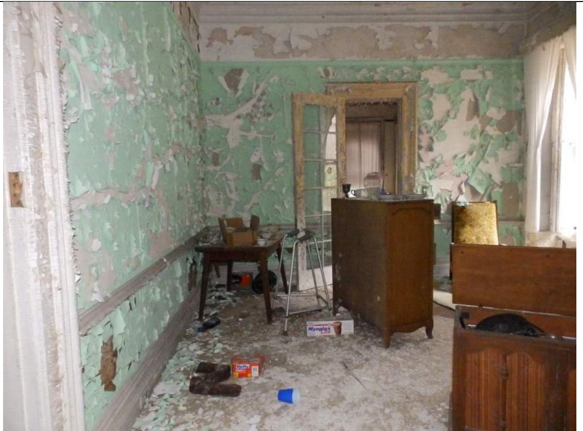
37. Room 103, looking north.
