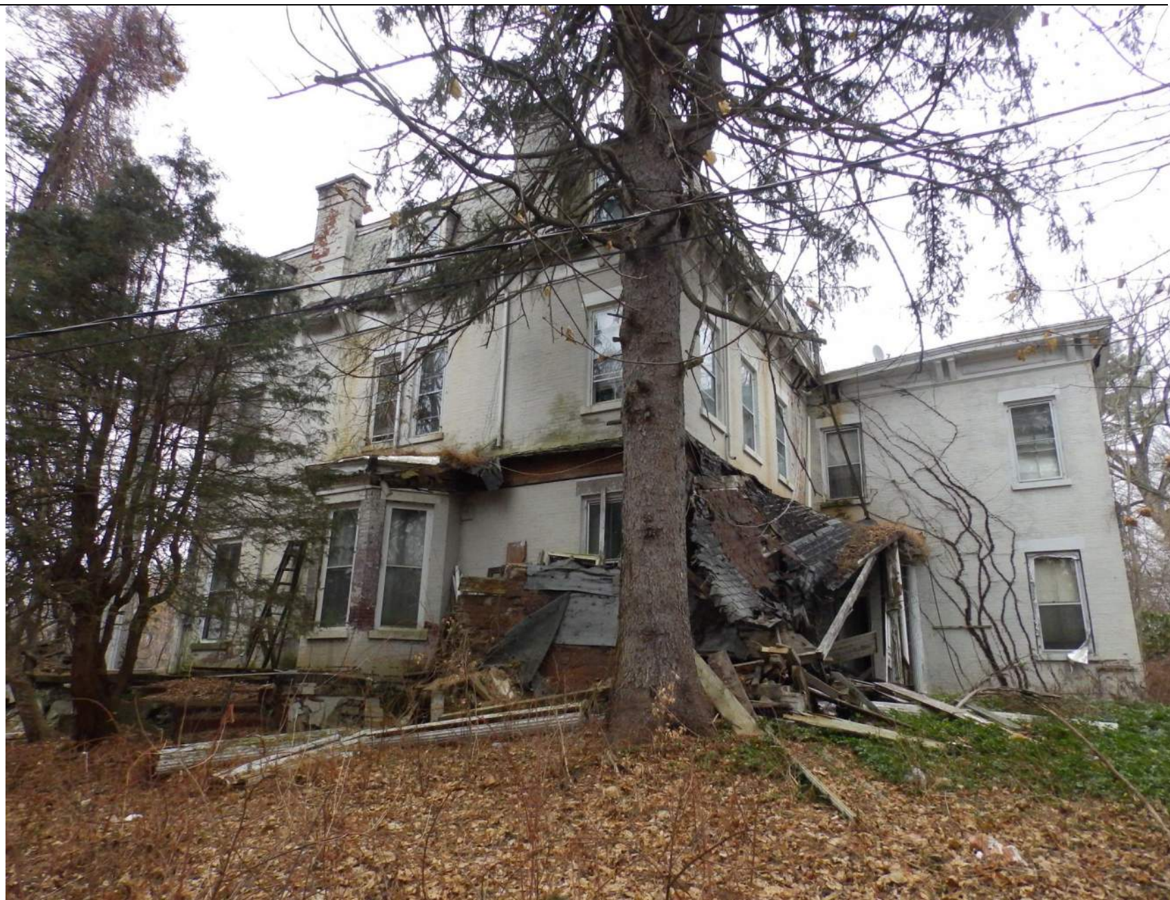
8. Oblique view of the western and southern elevations.
