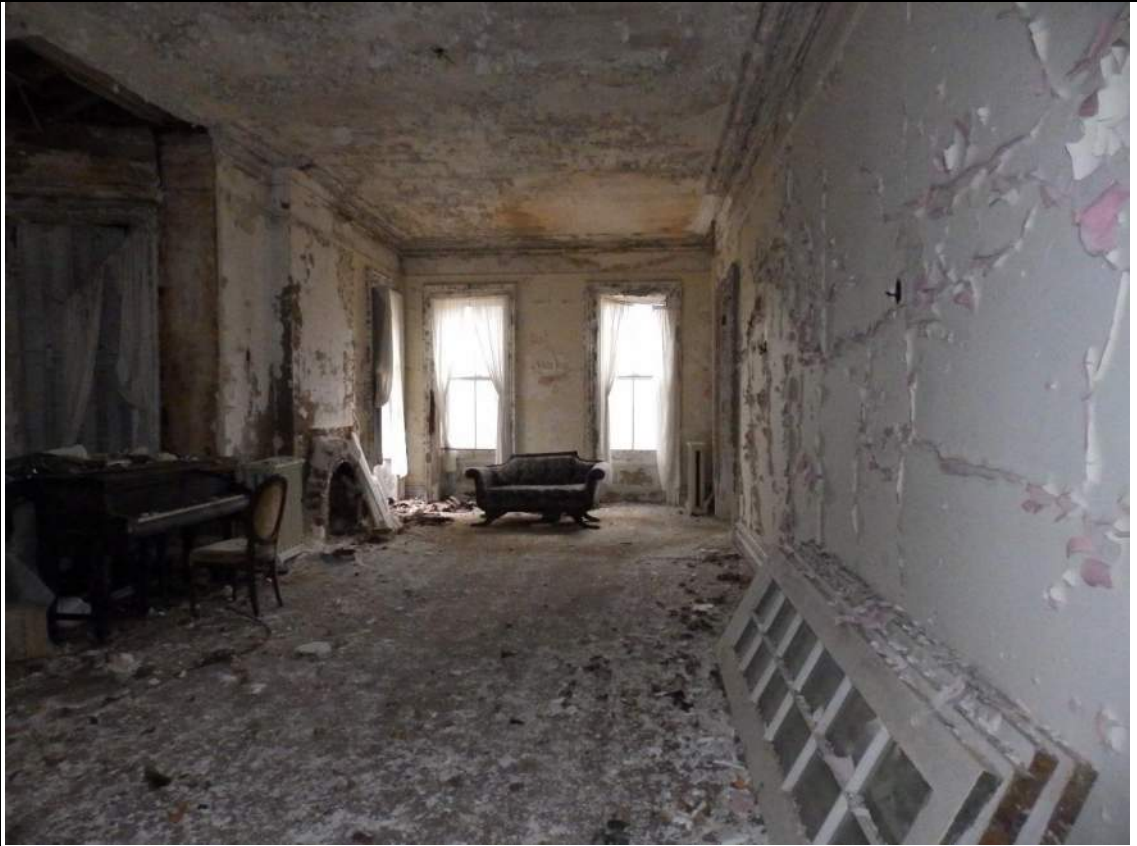
33. Room 101, looking north.
