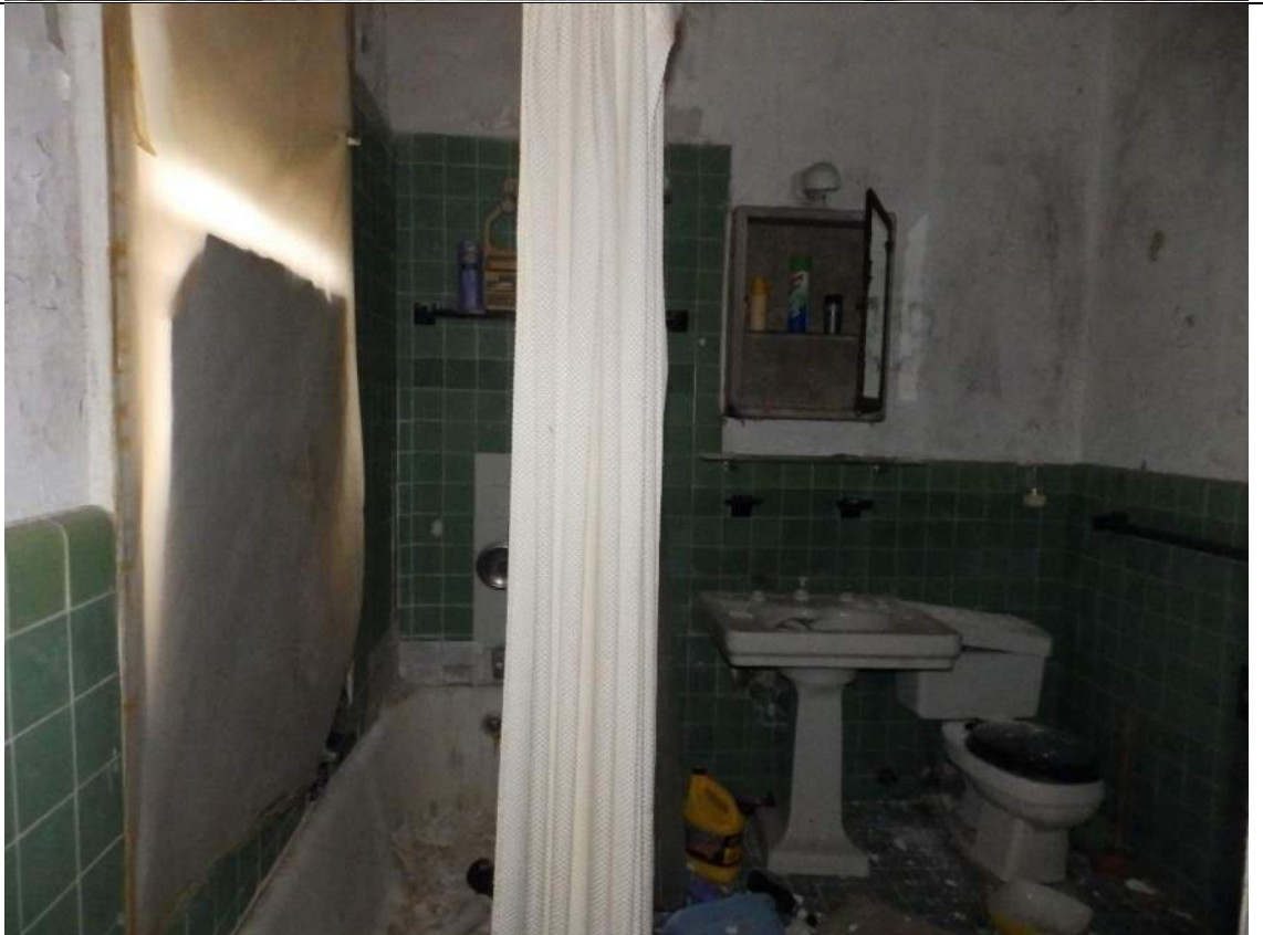
68. Room 211, looking north.
