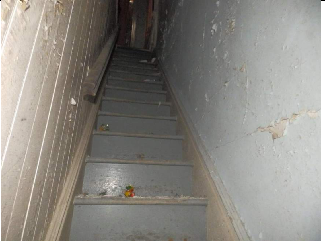
44. Utility stair to the area above kitchen.
