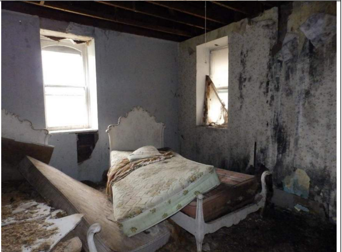
76. Room 303, looking southwest.
