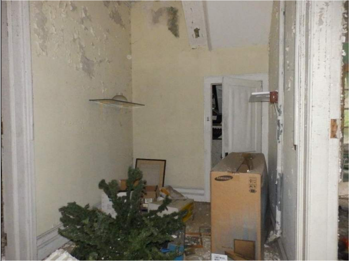
35. Room 102, looking north.
