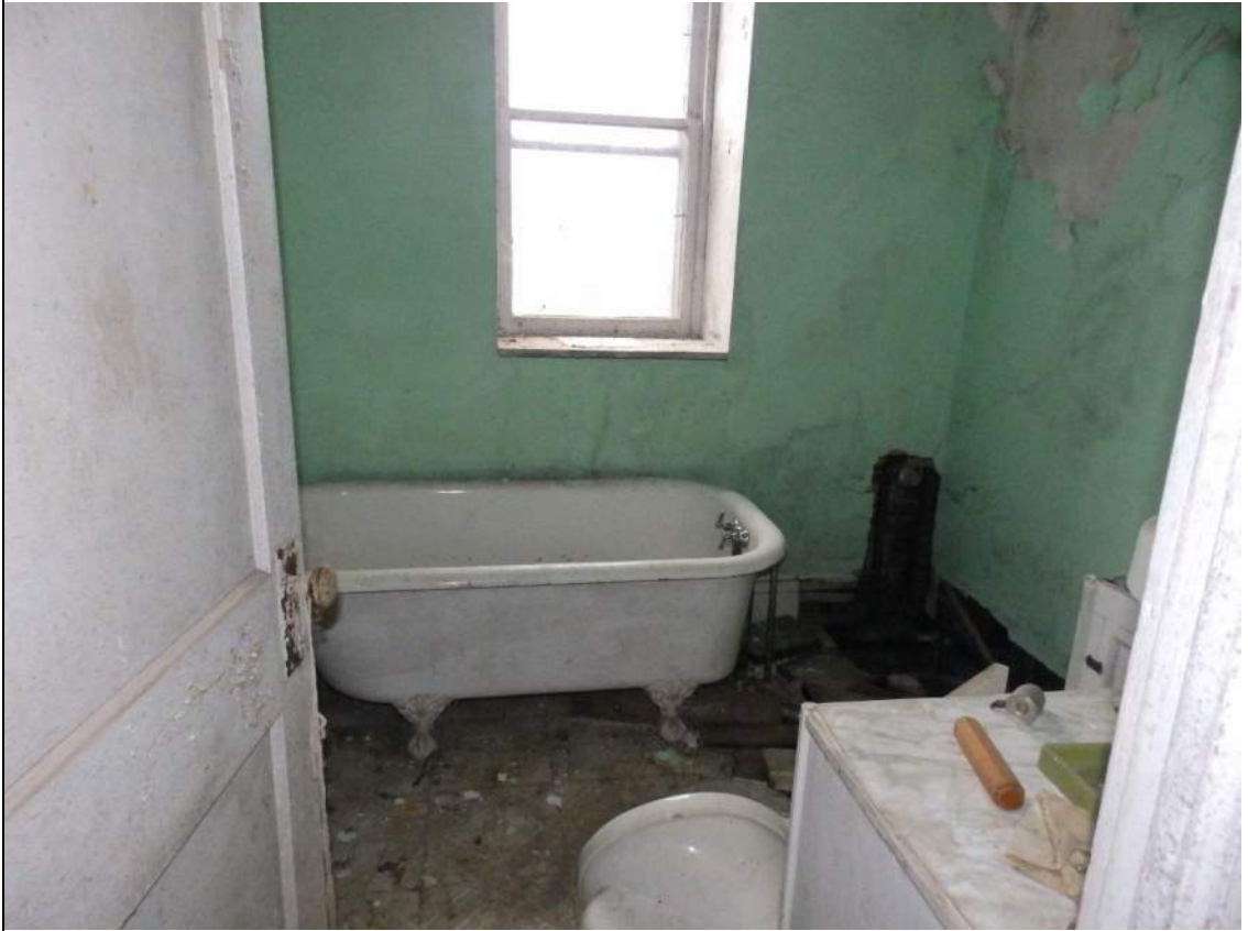
84. Room 310, looking north.
