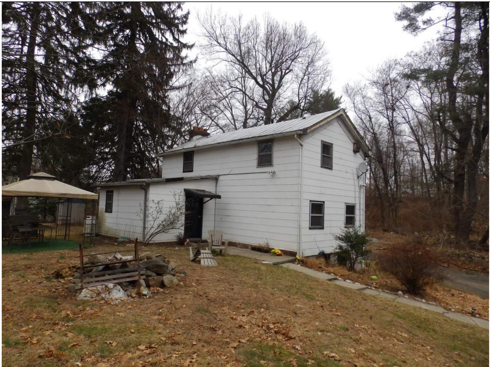
27. Oblique view of the western and southern elevations of the caretaker's house/
