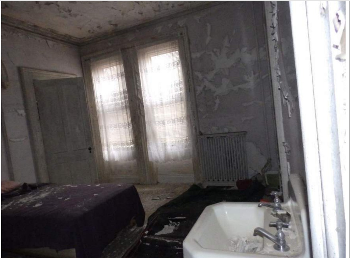
65. Room 209, looking southeast.
