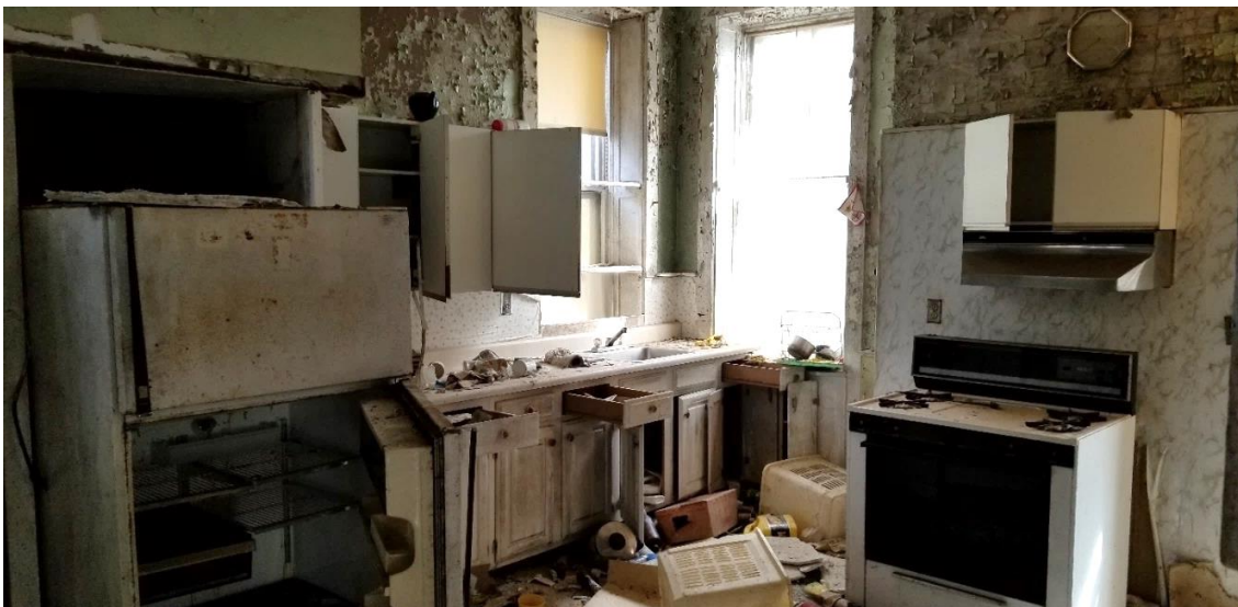
26. Kitchen – renovated after construction of structure
