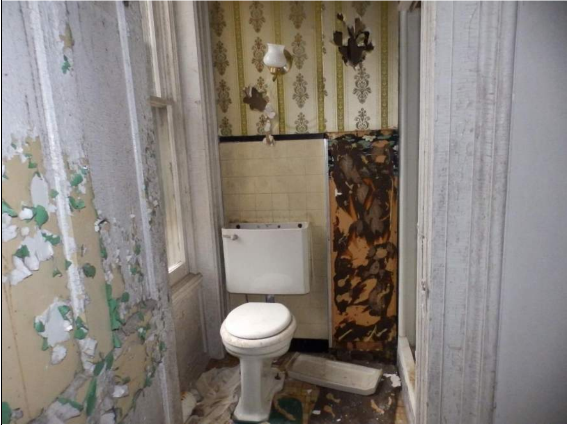
59. Room 202, looking north.
