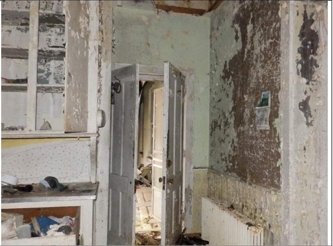
41. Room 106, looking northwest.
