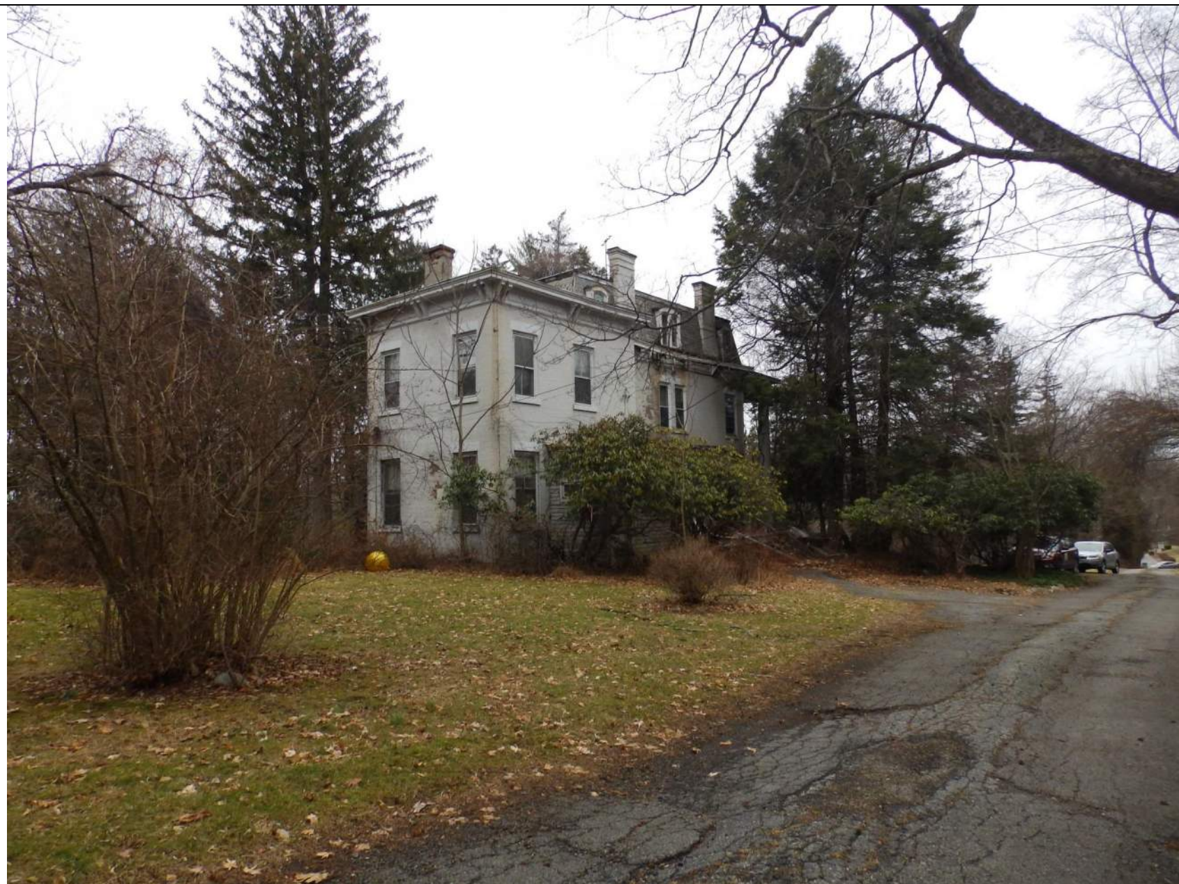
9. Oblique view of the southern and eastern elevations.
