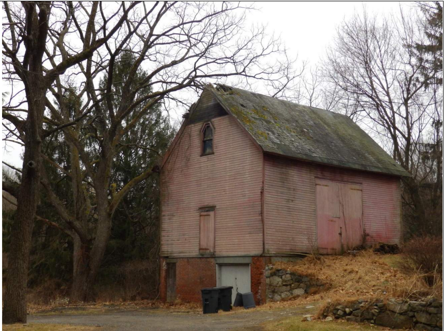
16. Oblique view of the eastern and northern elevations of the barn.
