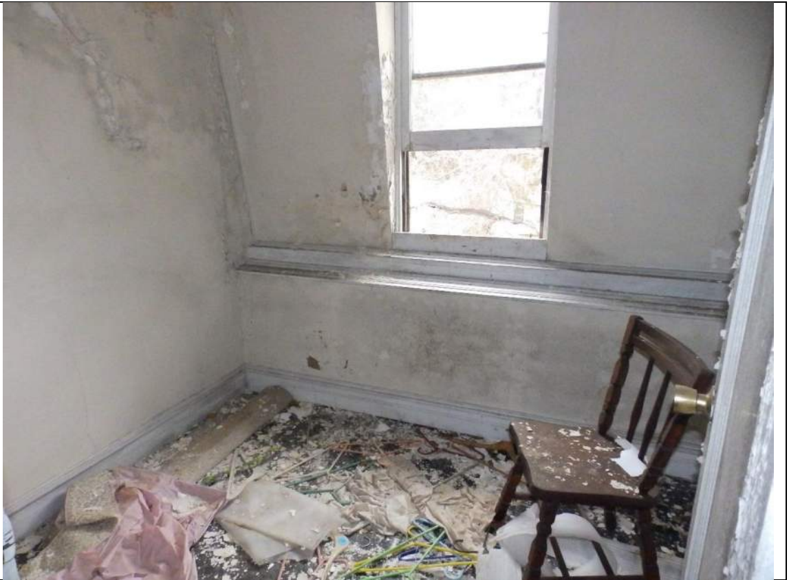
77. Room 304, looking south.
