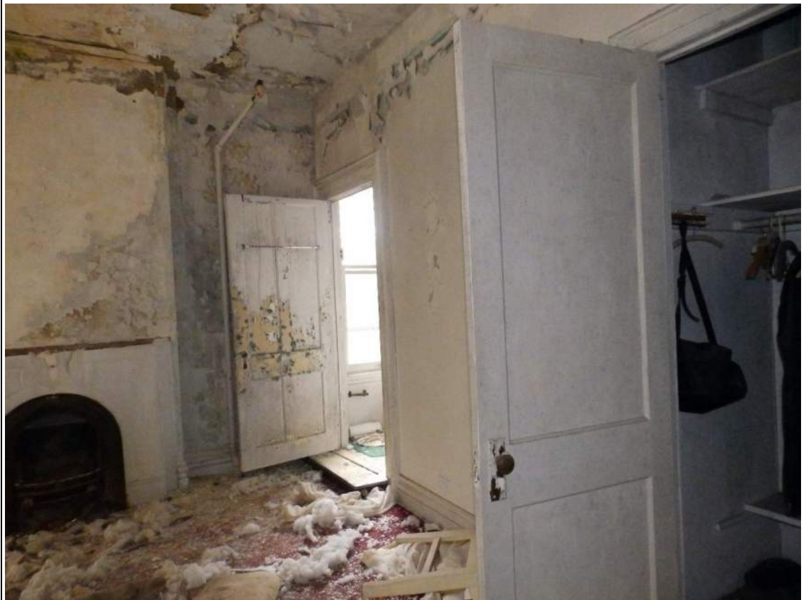
58. Room 203 looking west.
