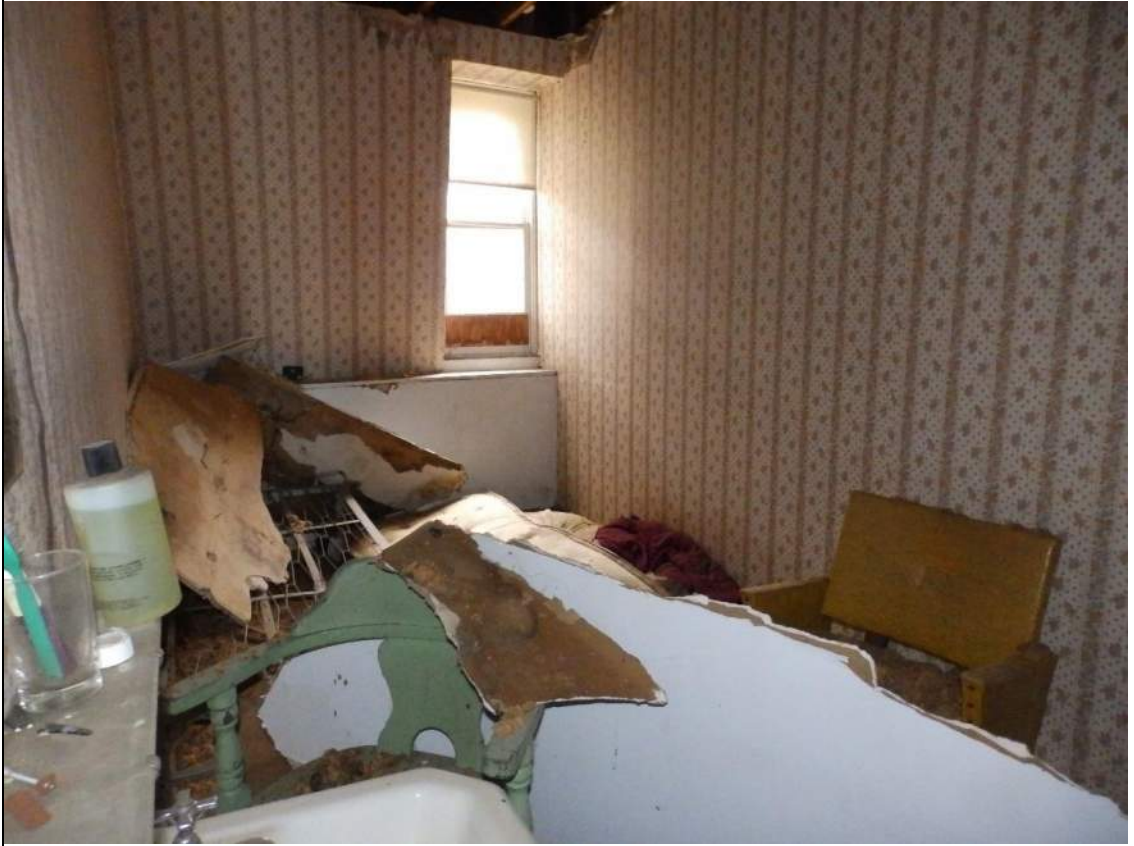
83. Room 307, looking east.
