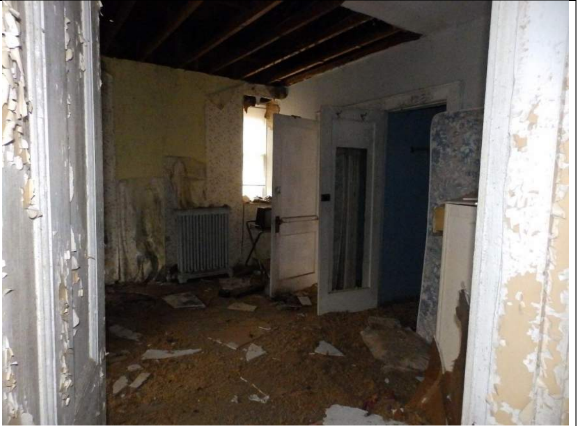
74. Room 303, looking northwest.
