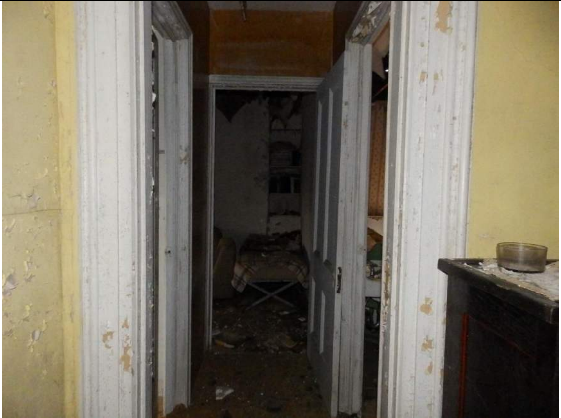
81. Small Hall to Rooms 307- 308.
