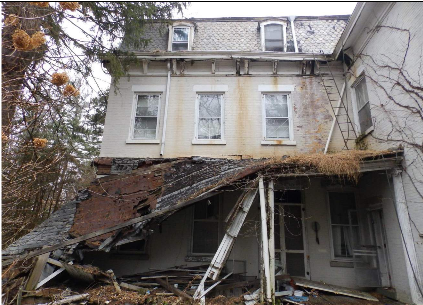
11. View of the southern elevation and rear entry.
