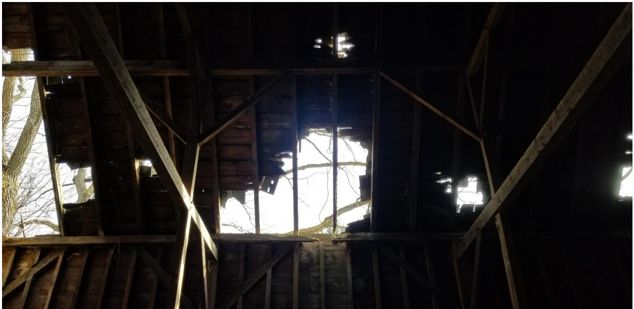
37. Damage and missing portions of existing roof
