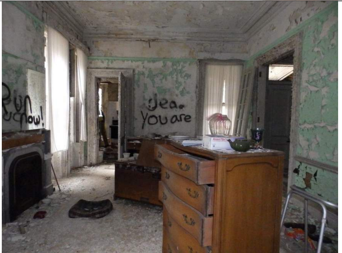
38. Room 103, looking south.
