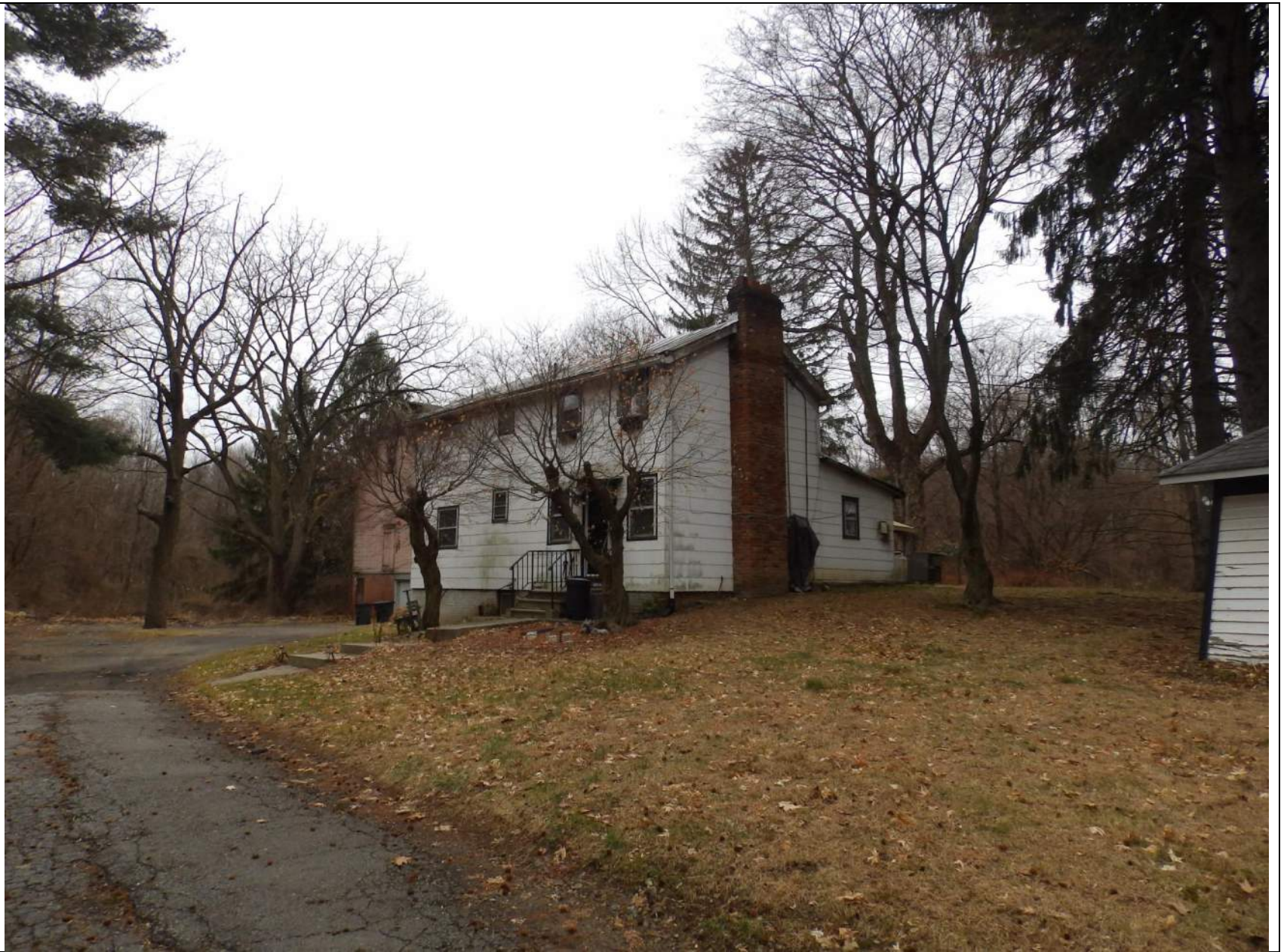
24. Oblique view of the northern and eastern elevations of the caretaker's house.
