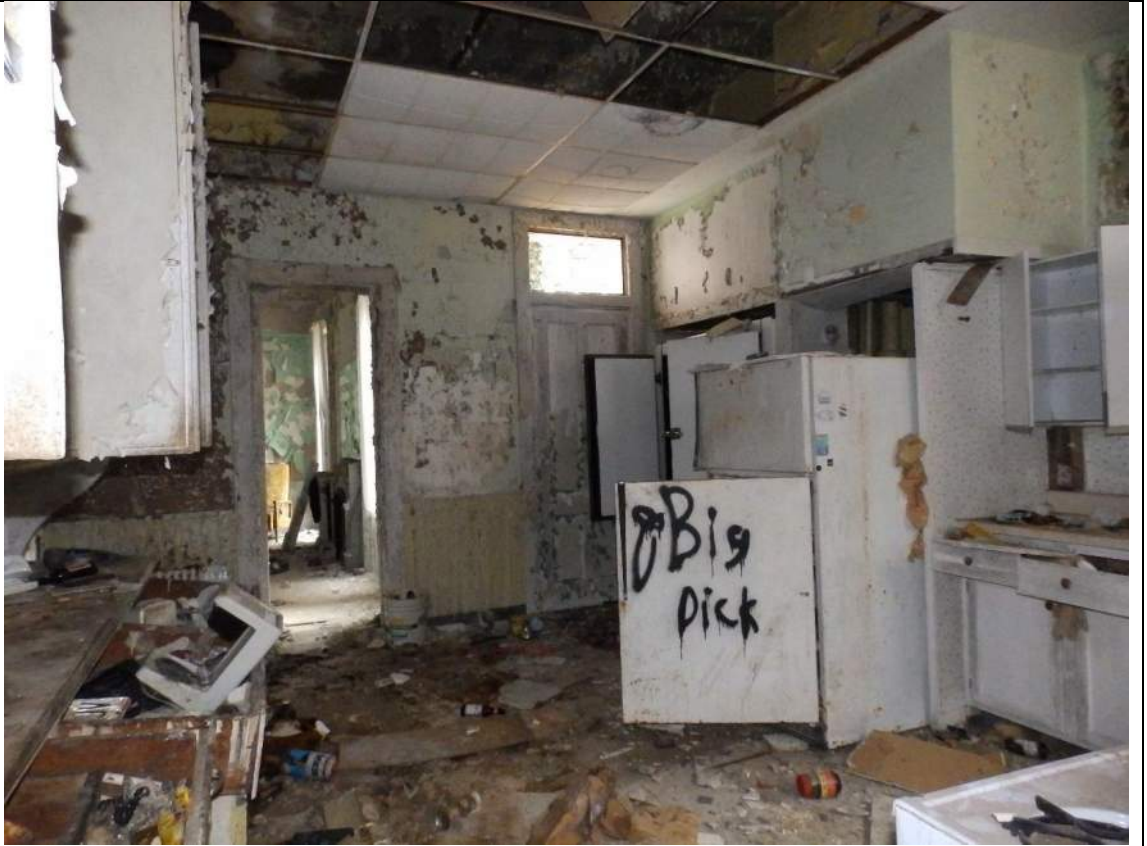
42. Room 106, looking north.
