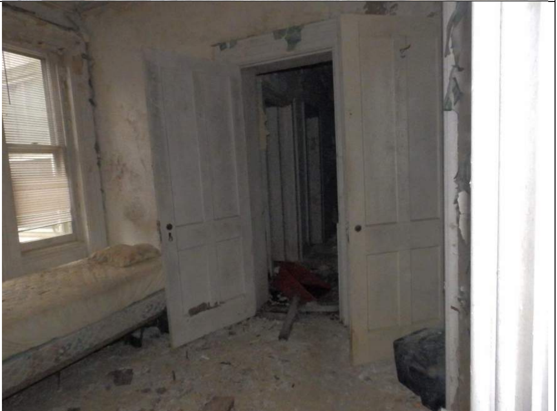
62. Room 205, looking south.
