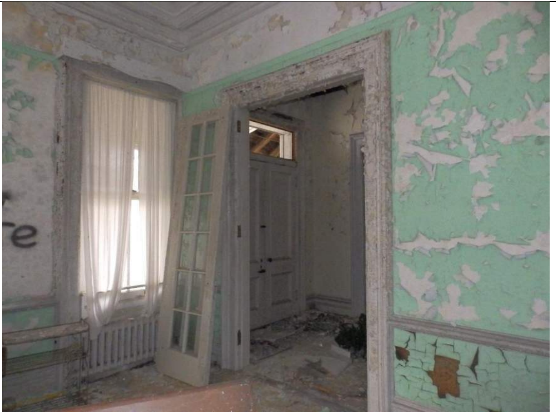
39. From Room 103 looking south to rear entrance.
