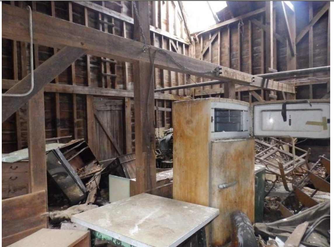
86. Interior of the barn, main level, looking southeast.
