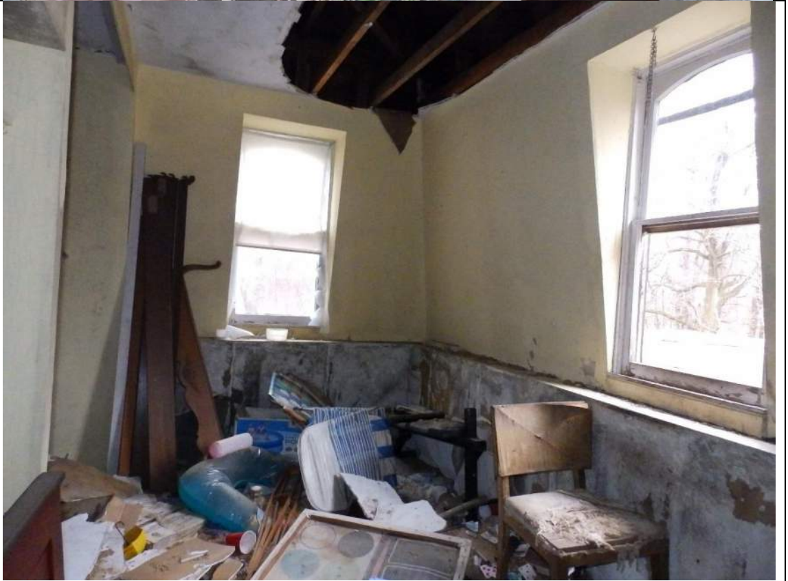
78. Room 305, looking southeast.
