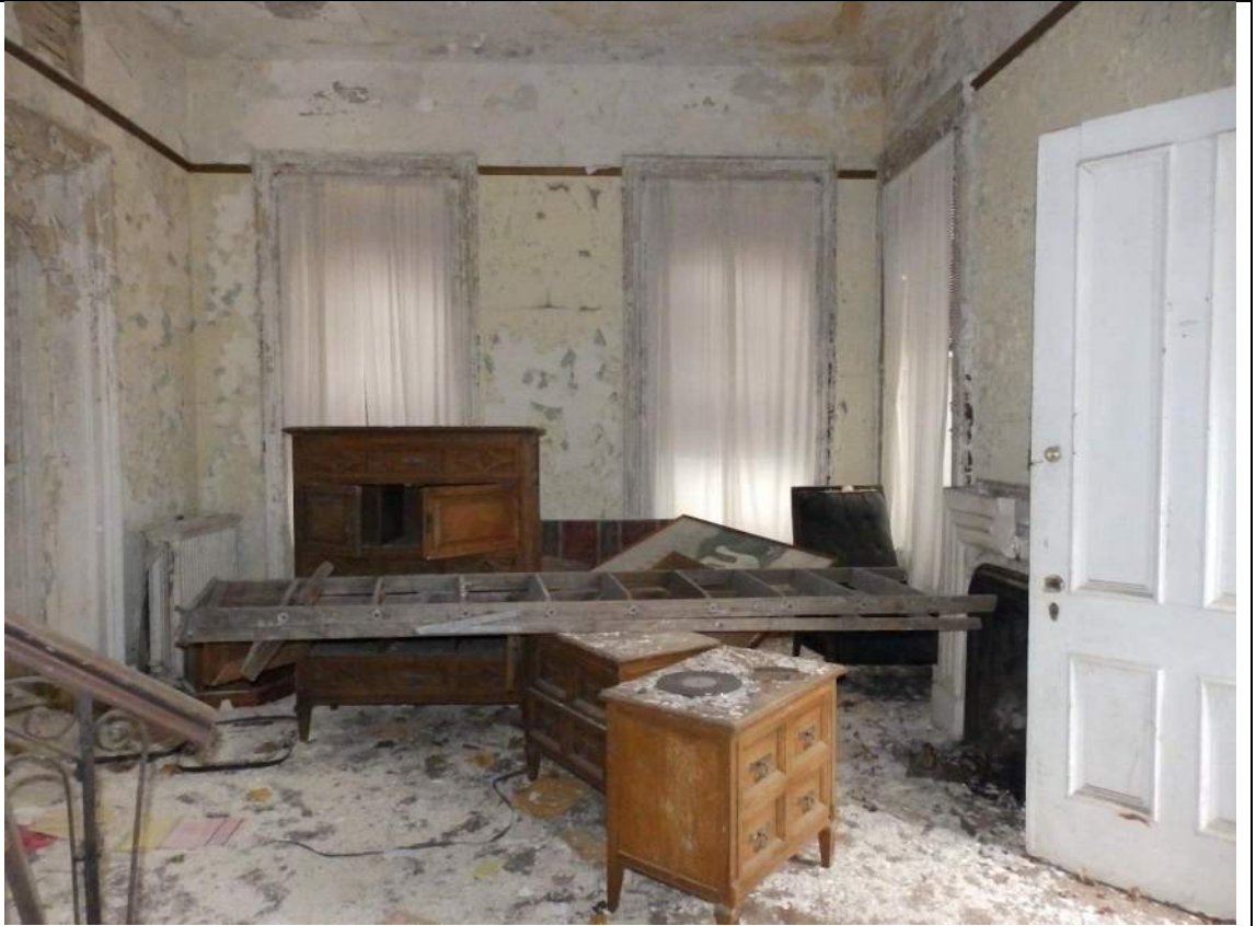
46. Room 104, looking north.
