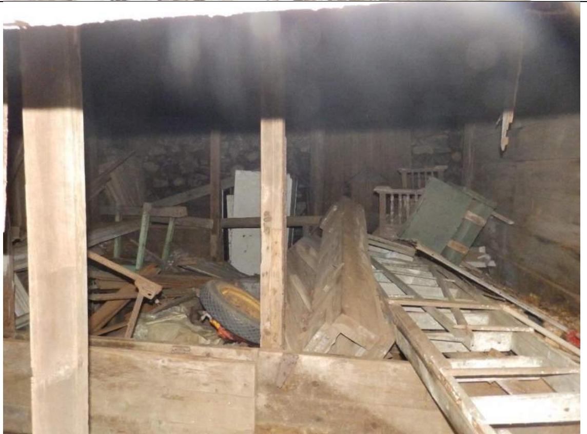
90. Lower level of the barn, looking west.
