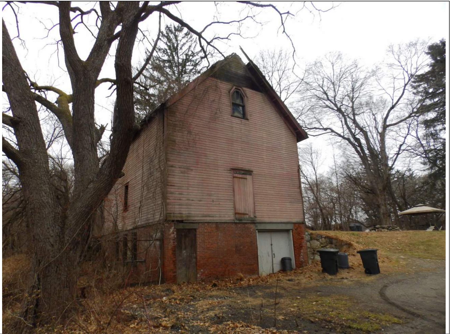
19. Oblique view of the eastern and southern facades.
